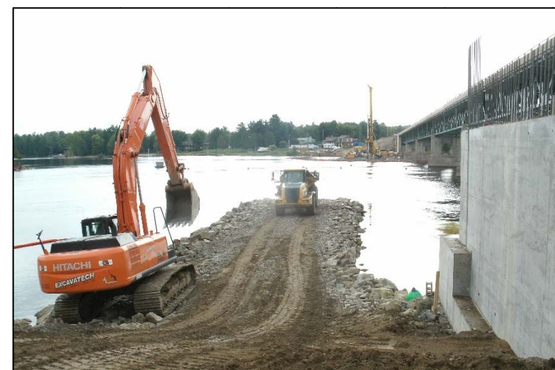
Figure 6.3.1: Construction of Causeway / Earth Berm (Des Allumettes Bridge)
