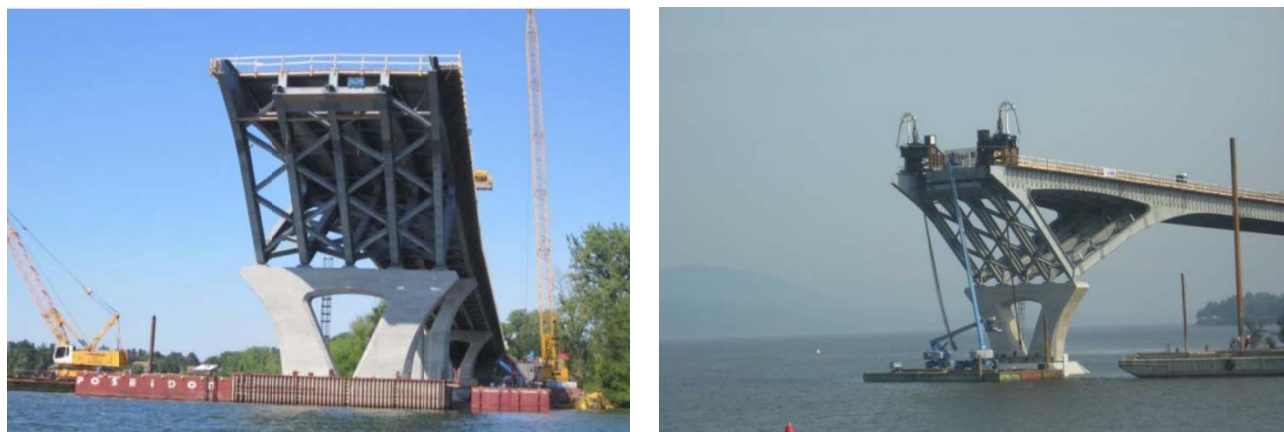
Figure 5.3.7: Steel V-Piers (Champlain Bridge)
