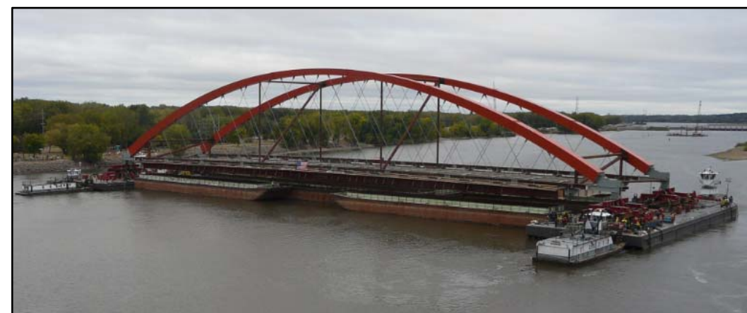
Figure 8.16.6.1: Erection of Hastings Bridge Using SPMT
