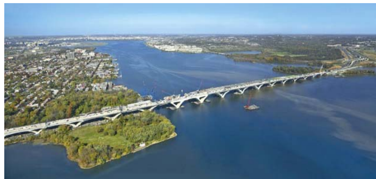
Figure 5.3.8: Concrete V-Piers (Woodrow Wilson Bridge)
